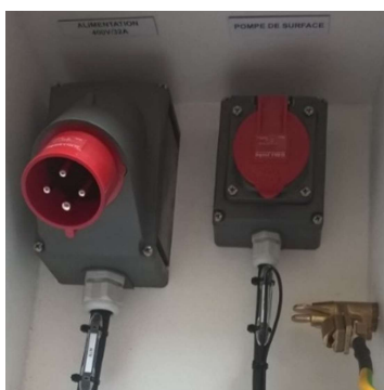
Figure 3: Alimentation générale non raccordée
