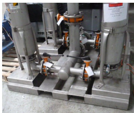
Figure 3 - Passage de fourches
